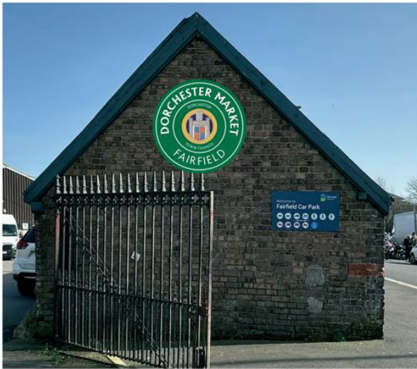
1. Fairfield Road/Maumbury Road entrance, South Lineys gable: 1200mm Ø
