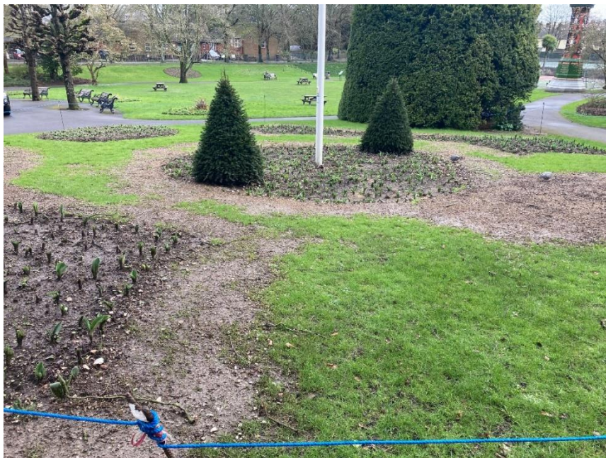
Completed levelling works Borough Gardens
