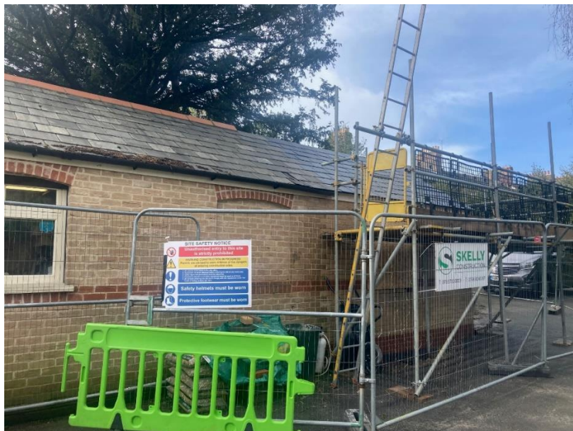
Mess room extension Borough Gardens, external works nearing completion.
