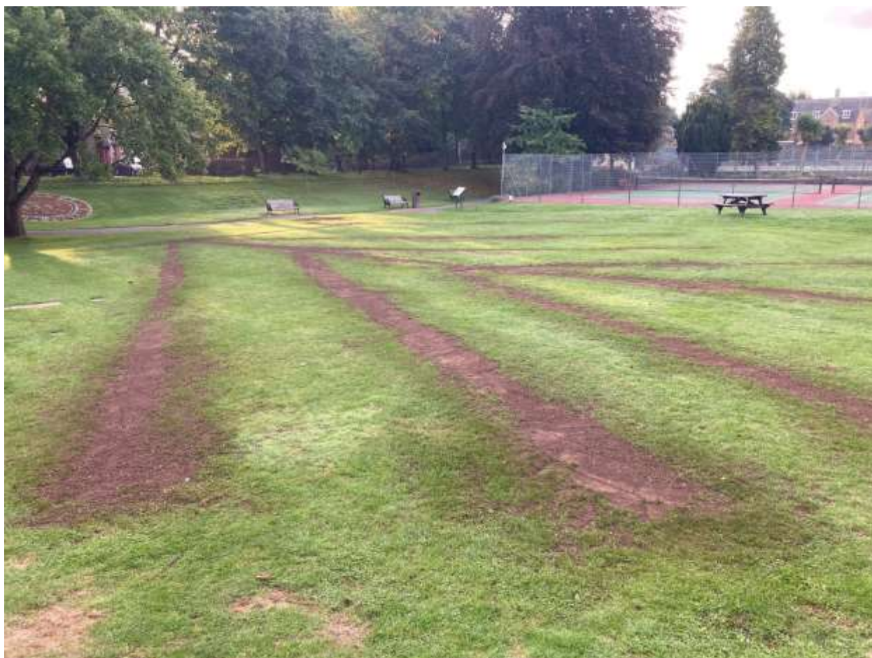
Recent topdressing works to sunken and droughted drain lines Borough Gardens.
