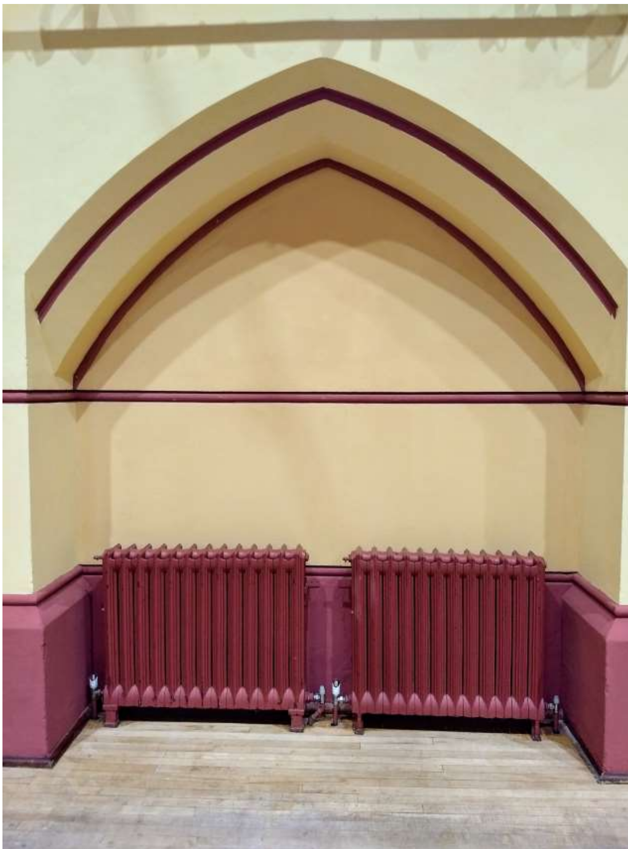
Lower walls being painted
