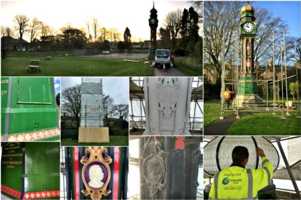
The above is a montage of the works to the clock and it shows very well the improvement from its previous condition and how shiny the new coating is.
