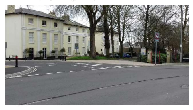
Junction after access improvement works, note wider footways, paved entrance, raised table and narrowed road width.
